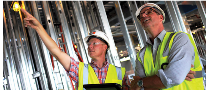
Project Superintendent Tom Owens (left) takes President/CEO Glenn Granger on a tour of a project site. Owens and his crew on site implemented the use of PlanGrid, an intuitive, sheet-based mobile construction app that keeps everyone building from the most current set of drawings.
